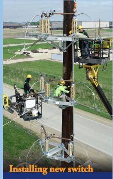
**Above** Corn Belt Power transmission crews install a new two-way switch pole outside the Whalen Substation May 18. The new substation will help power Shell Rock Soy Processing inside the Butler Logistics Park.
